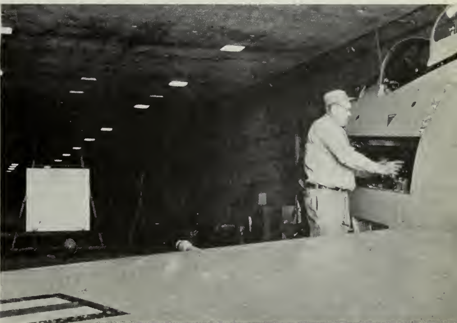
SHOOTING THE WORKS —Armament Test Division puts naval aircraft fire power to the test. Here an FJ-4B Fury is bore-sighted in division's firing tunnel.
